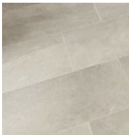
Floor Tile + Shower Walls: DT Slate Attache SA06 Meta Gray 12x24 Laid horiz.
